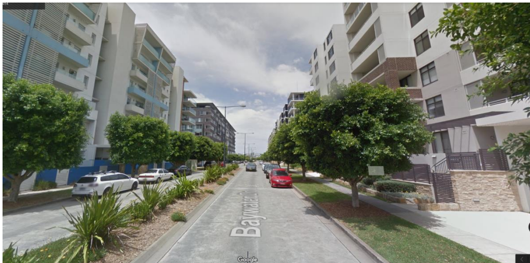
18. Example Residential Development with open street feel, Wentworth Point Source: Google Maps Streetview
